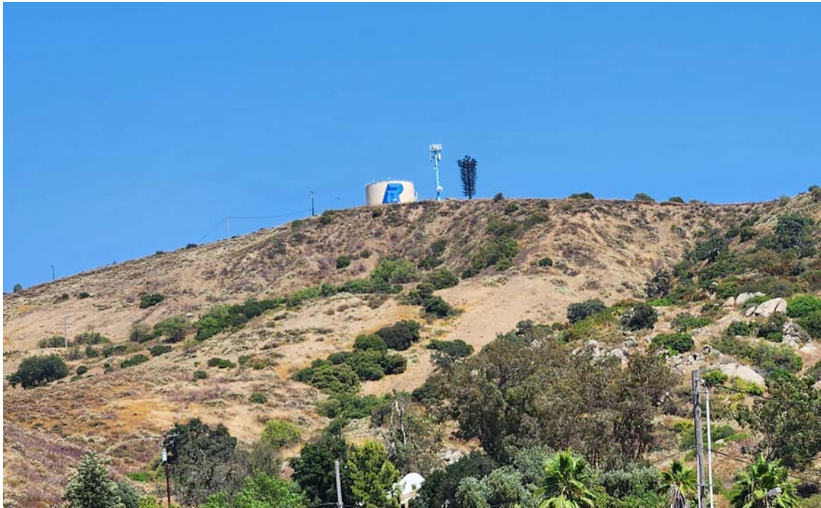
View of Robinson Tank from Hanson Lane. Photo courtesy of RMWD.
